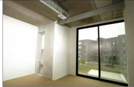
The Spancrete Wall Panels were left exposed to give the Row Houses a post-modern urban feel.
